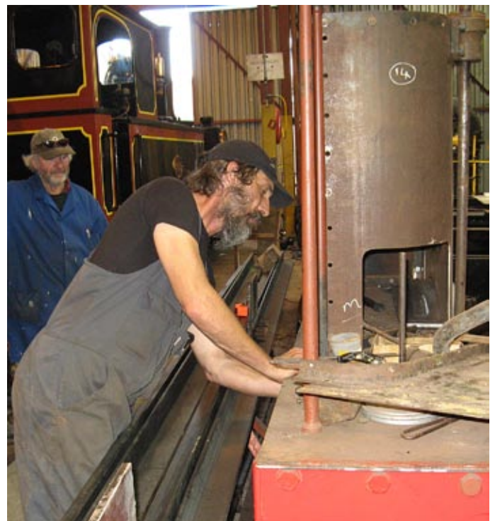
ABOVE: Paul Spearpoint, watched by Dave Lye, works on the fireman's side coal bunker on April 28 2009.
