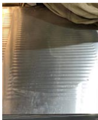
ABOVE LEFT: One of 21's original corrugated aluminium wall panels with post service garden shed green paint.
